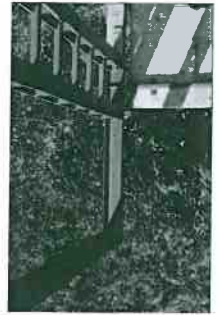
STEEL FRAME CANTERLIVER WITH TIMBER STRUCTURED ROOFING
